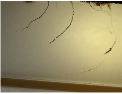
Cracks under shelving unit. Otherwise good condition
