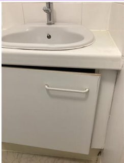
Cracked unit under wash basin
